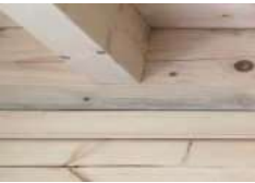
Timber turning grey and blue
